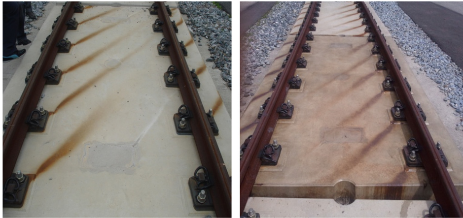
Fig. 3. Concrete slab track, before (L) and after (R).
